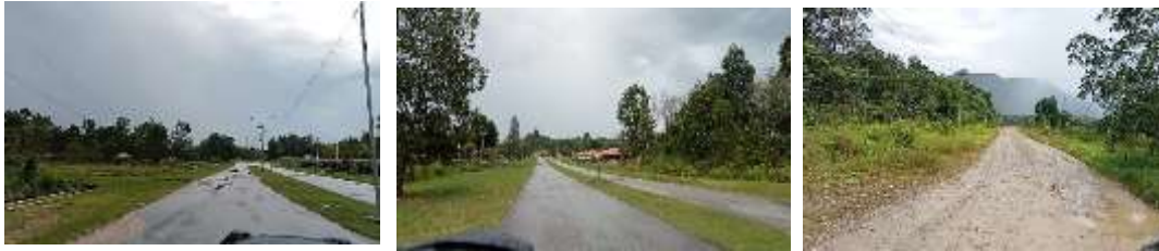
Figure 2. Road Network Conditions
